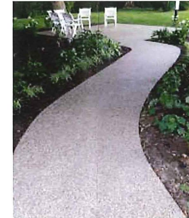
EXPOSED AGGREGATE PATH
