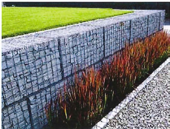
GABION BASKET DARK STONES
