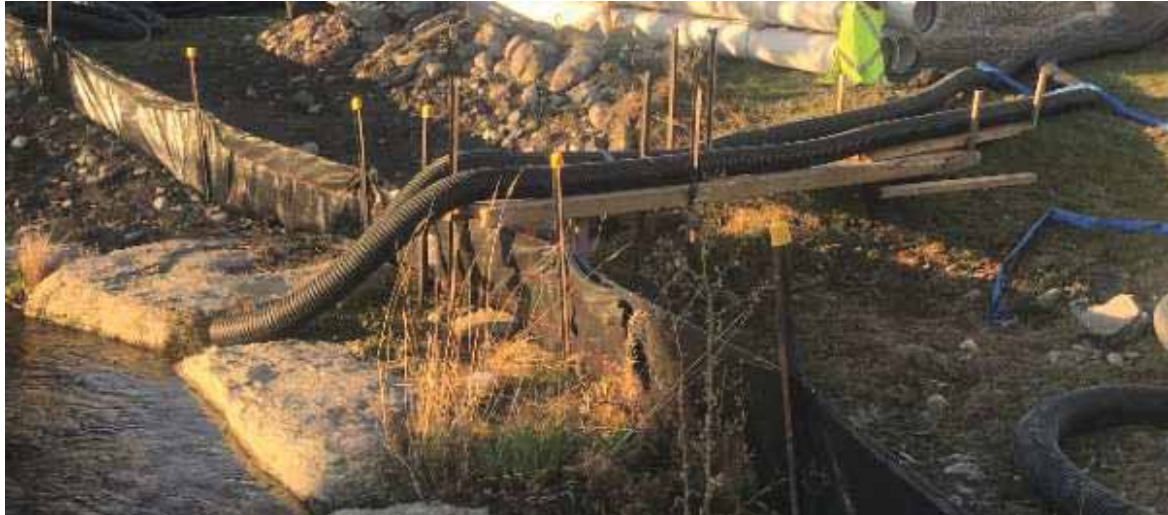
Figure 5: Example of Novacoil supported by timber bridge span (Source: Author's collection)
