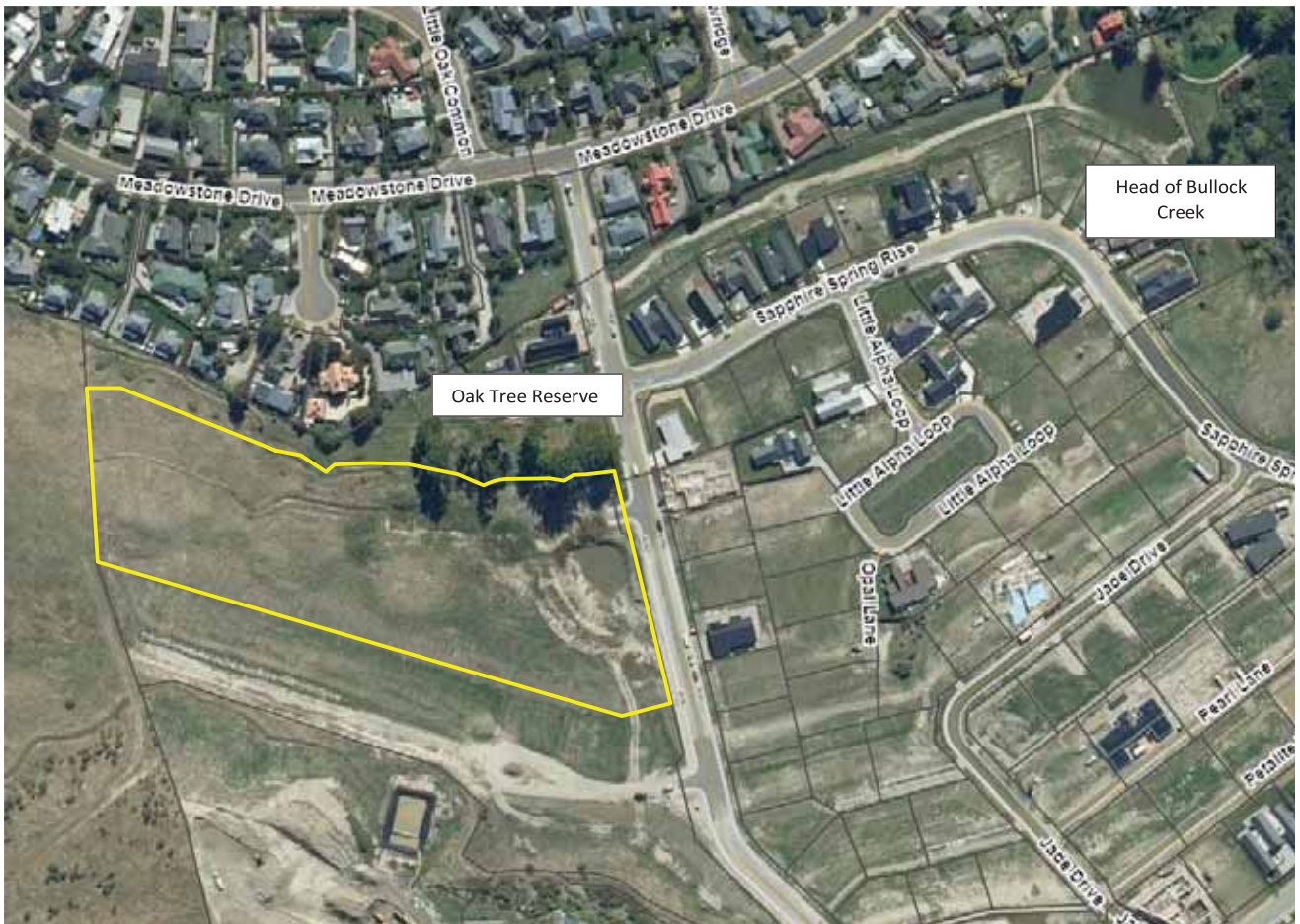
Figure 1: Aerial view of Stage 4 site and key environmentally sensitive locations and receptors
