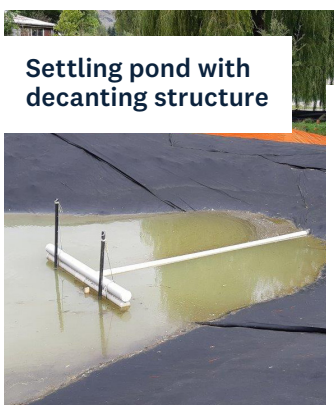
Sediment sinks to bottom leaving only clean water on top.
