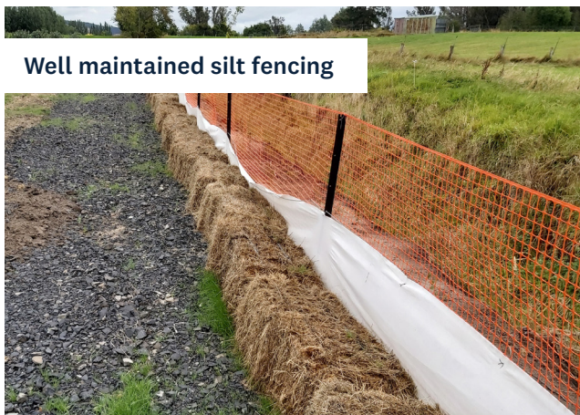
Artificial covers may be used to filter sediment and cover exposed soils.
