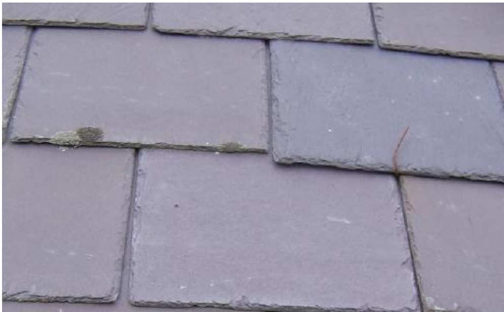
Figure 21: Misaligned slate
