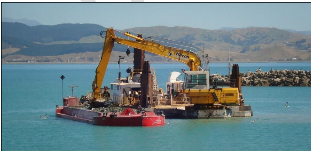
Figure 3-3: Typical backhoe dredge loading a barge
