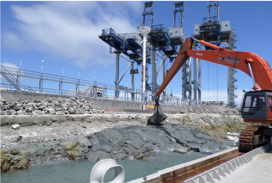
Figure 3.12: 70 Tonne Longreach Placing Mudcrete at POAL Reclamation
