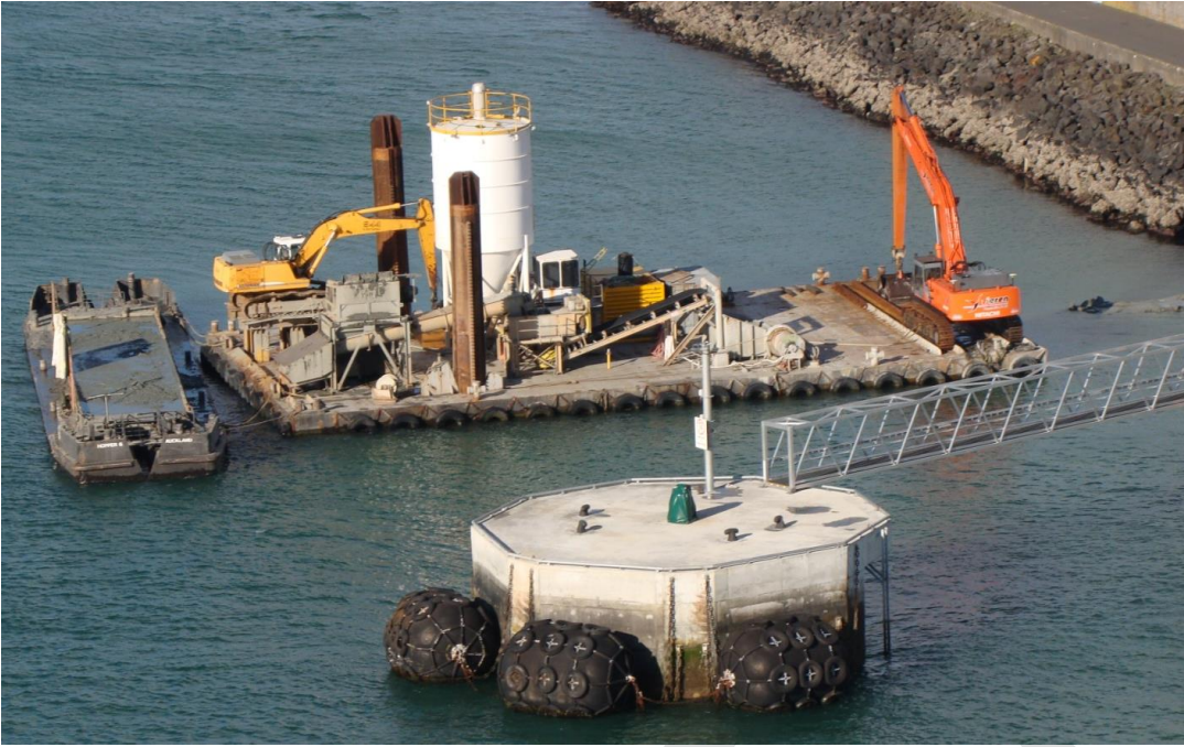
Figure 3.11: Pugmill Barge Mesenge Working on POAL Fergusson Reclamation
