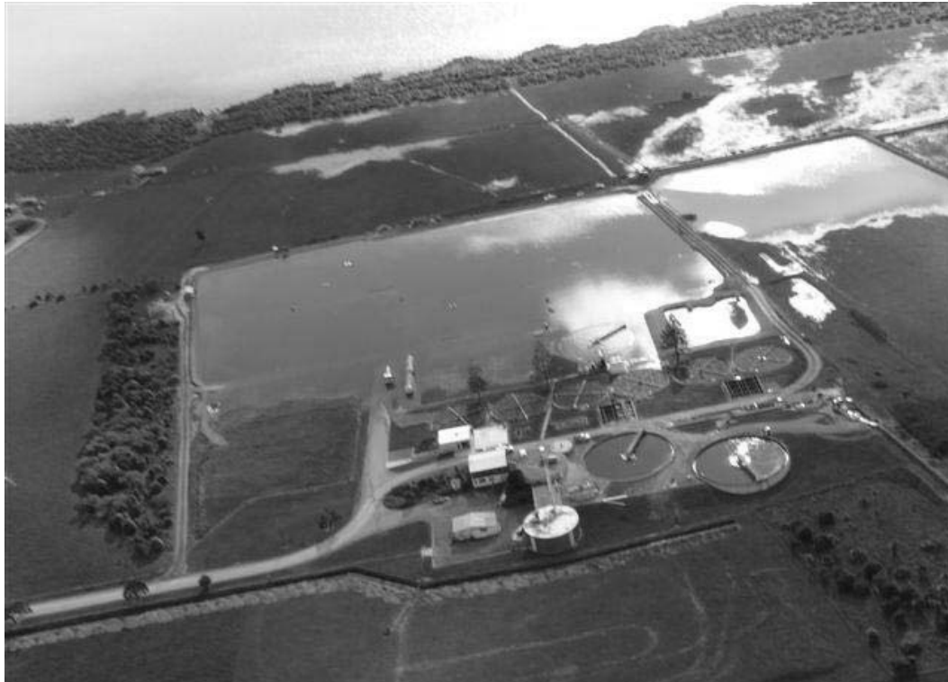
Overflow of effluent from the treatment plant, August 2008
