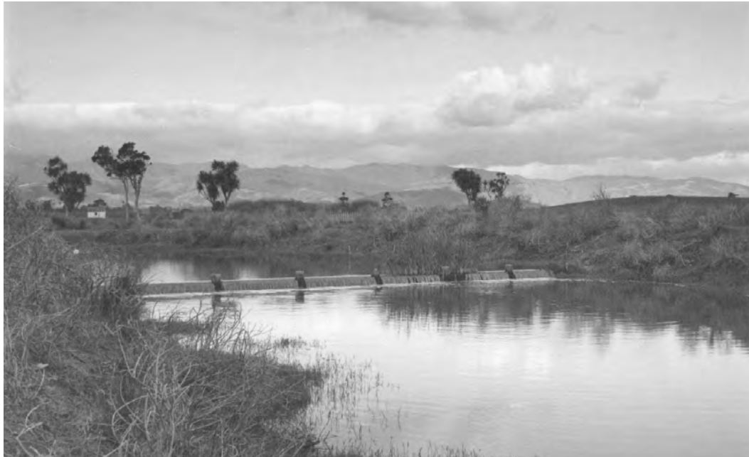
Photograph of the concrete control weir at the outlet of Lake Horowhenua, 1977
