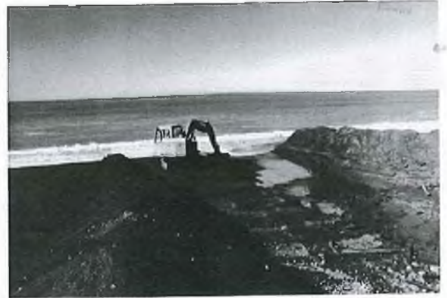
Toro Waaka photo 2: Digging out the Bar at Mohaka Beach/River Mouth 1993
