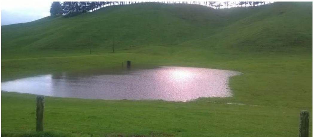
Photo 8 – Shows the detention bund in Photo 7 capturing water.
