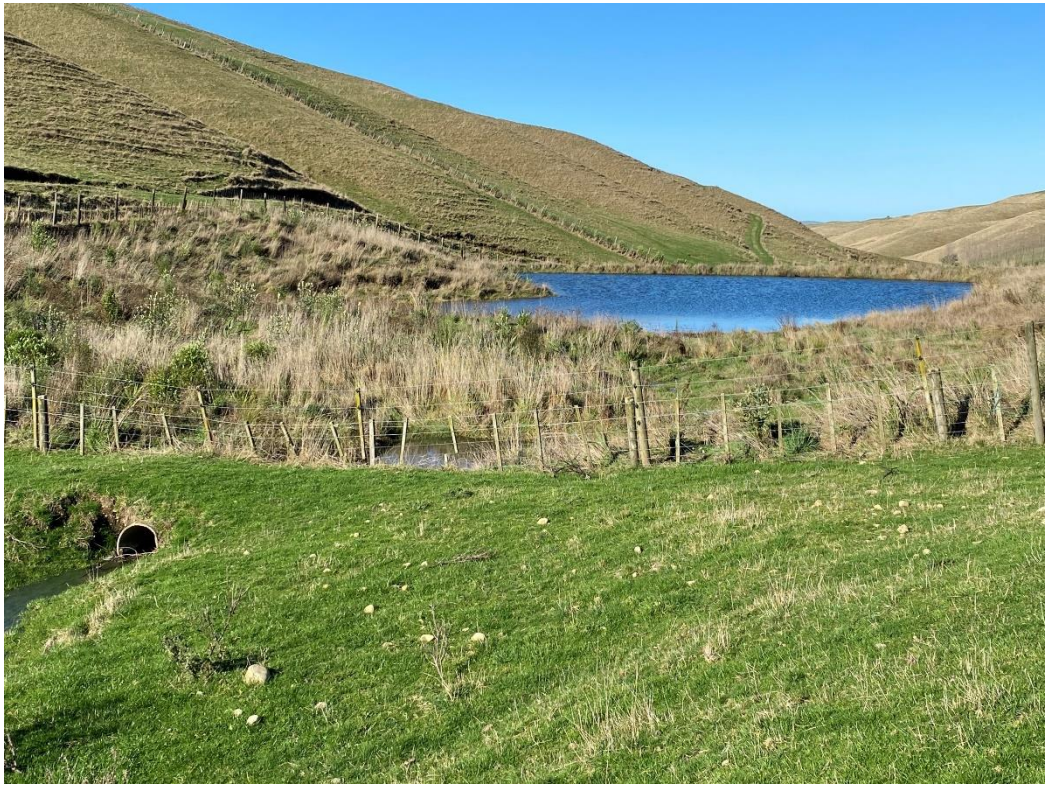
Photo 1 - Sediment traps are best situated in the critical source area where water naturally flows. They can range in size from large ponds to small scoops out of the ground.
