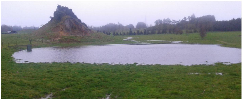
Photo 10 – A Detainment Bund starting to fill during a run-off event. Lake Rotorua catchment.
