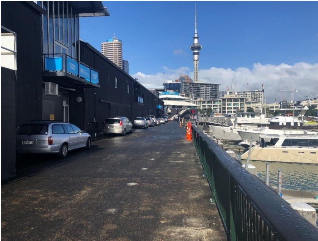
Figure 14: Existing western side of Hobson Wharf
