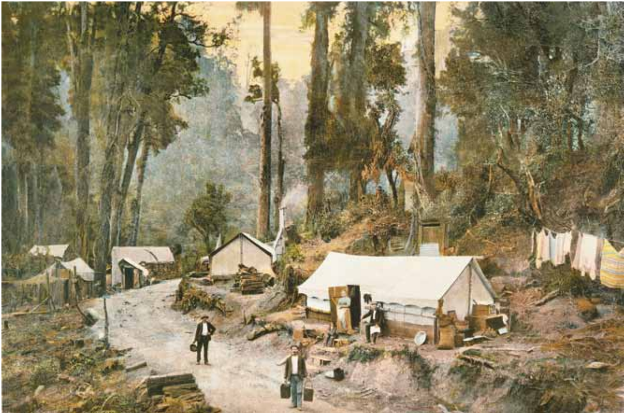
Camp life in the New Zealand bush, 1908. Railway workers on the North Island main trunk line, dwarfed by tall trees near the Hapuawhenua Viaduct, north of Ōhakune, where workers toiled in harsh conditions amid noise and smoke.
