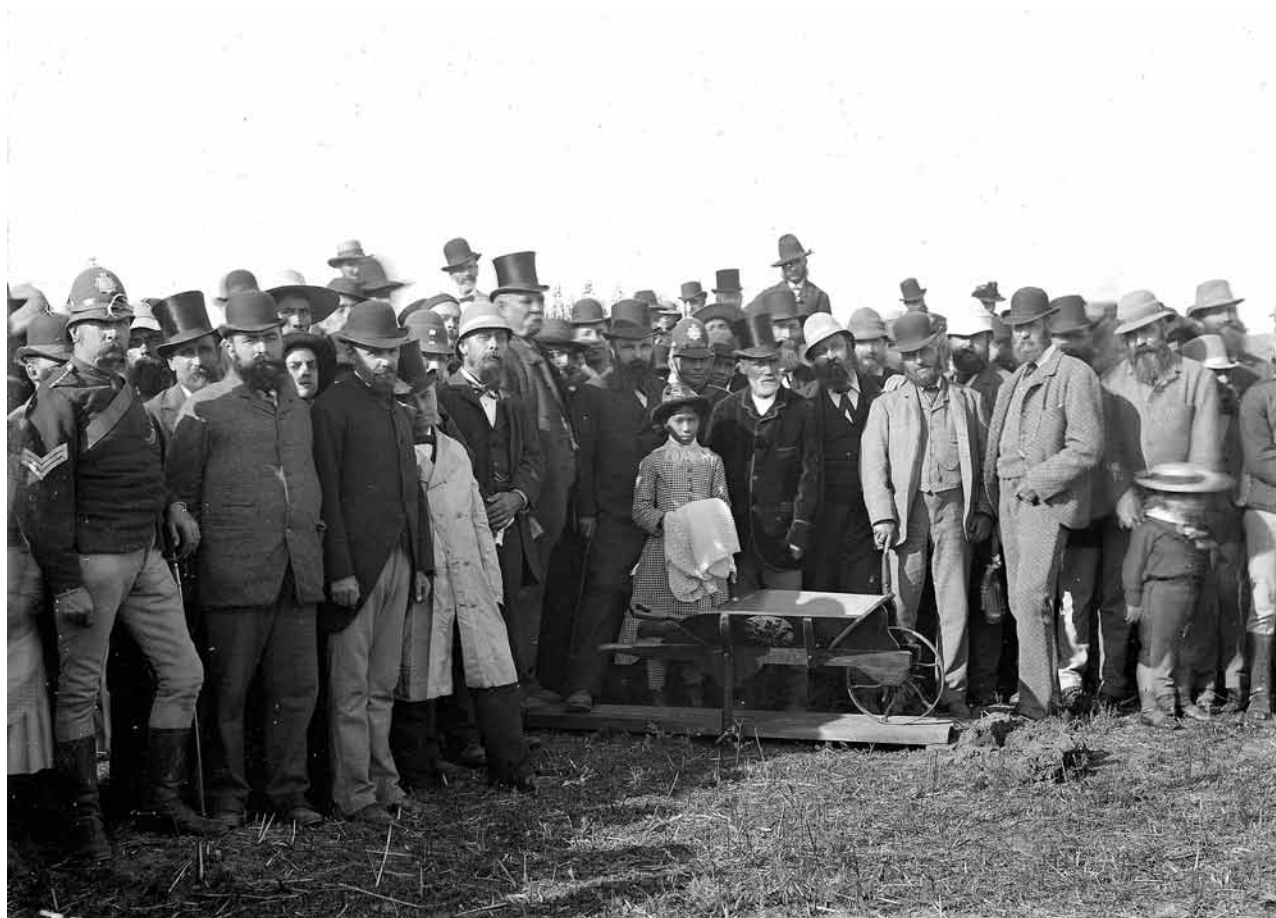
The first sod is turned for the main trunk railway, 15 April 1885. The group, which includes Rewi Maniapoto and Sir Robert Stout, is standing on the confiscation line at the southern bank of the Puniu River.
