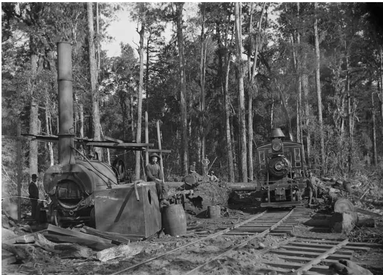
Climax locomotive 898 hauling logs in the bush near Ōhakune. Rail was another means of transporting timber in the early 1900s.
