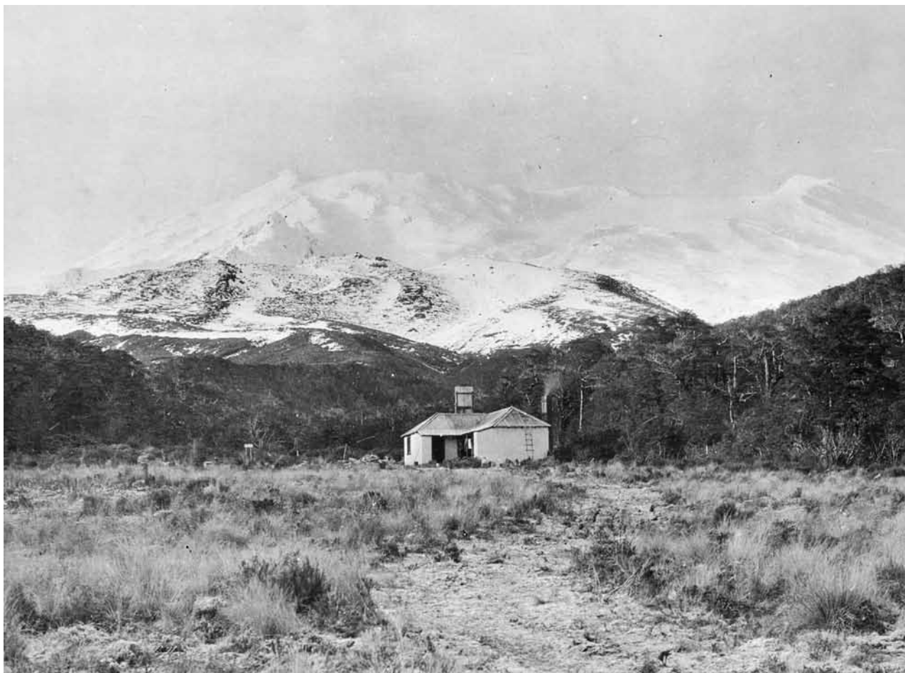
A cottage at Whakapapa built in the 1920s. Possibly one of the first to be built in the area to accommodate skiers, this house was followed by exclusive accommodation for ski clubs.
