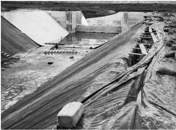
The butynol lining of the Te Whaiu Canal
