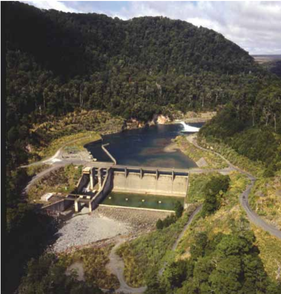
The Rangipō Dam
