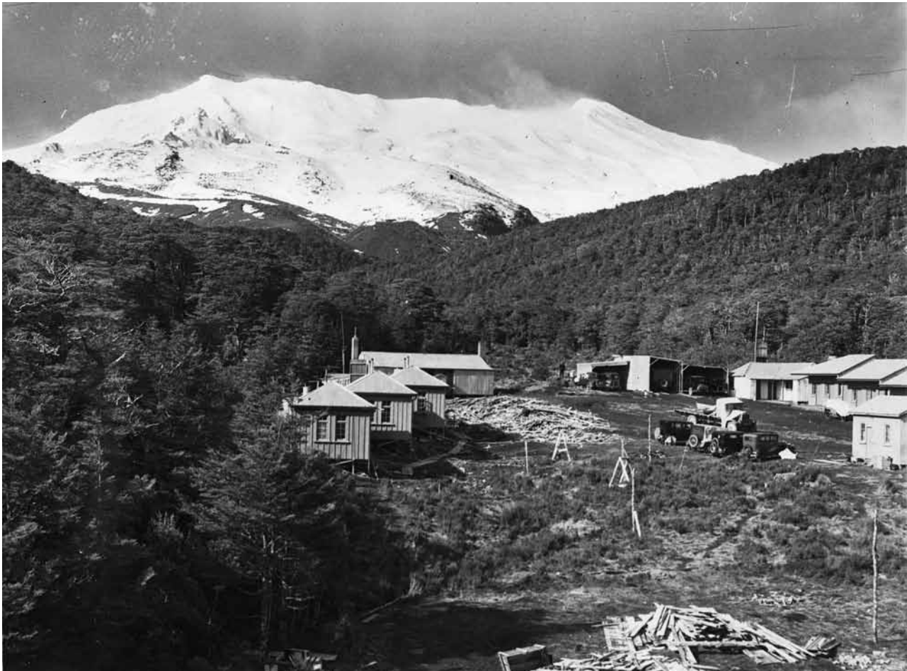
Accommodation alongside the Chateau Tongariro. In the 1920s and 1930s, outdoor recreation on Mount Ruapehu was aided by developments such as a camping ground and these huts, and these developments were instrumental in encouraging young people to visit the park.
