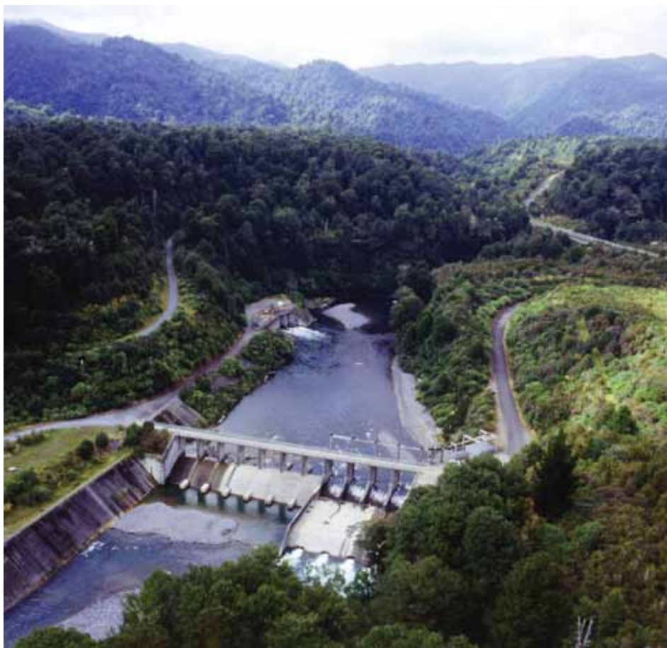
The Poutū Canal and Dam. The construction of the dam altered the environment so much that spawning areas for trout were lost.
