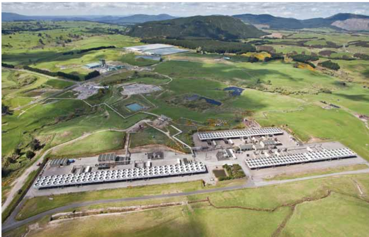
Geothermal power station at Mokai, Taupō. Behind the station are glass houses, a dairy factory, and a worm farm.
