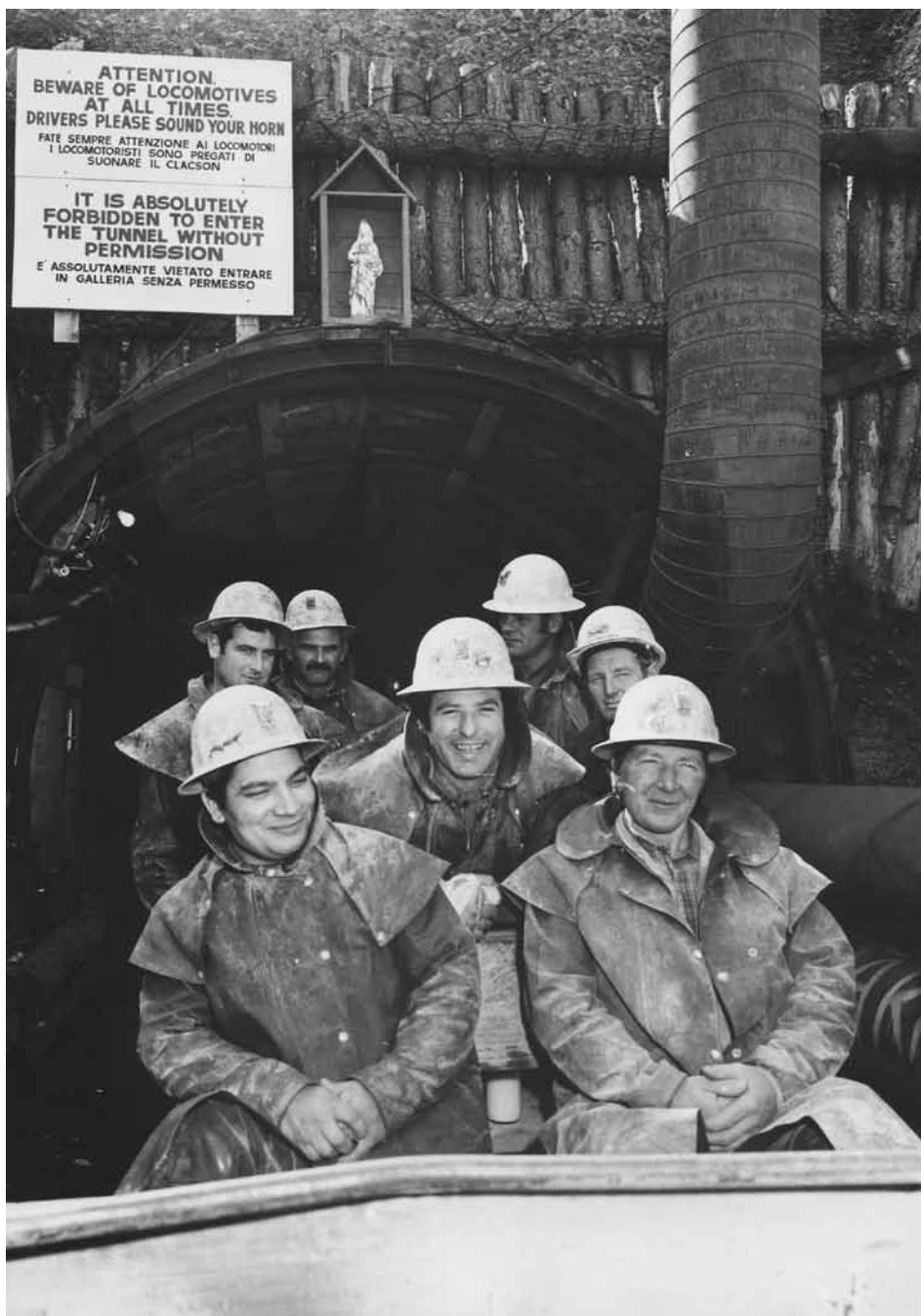
Italian workers on the Tongariro power development scheme. The Italians were brought into New Zealand for tunnelling work. Camps were established at each end of the tunnel, as well as where the two sections met.
